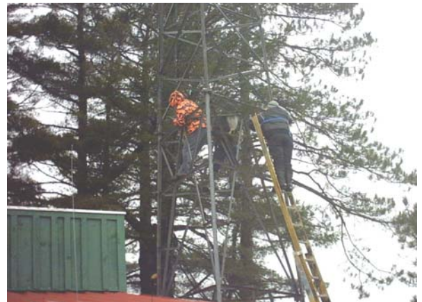
Above – Rich looks on as the tower top is raised Below – Mike, Tony & Rich bolt the sections together
