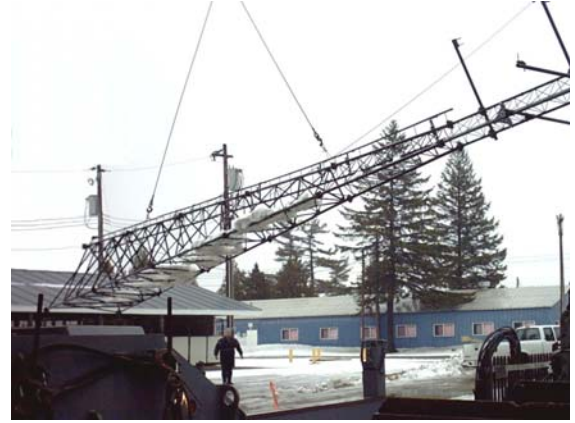
Above – Rich looks on as the tower top is raised Below – Mike, Tony & Rich bolt the sections together
