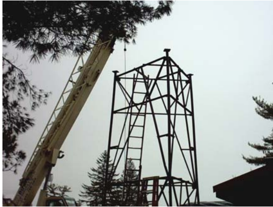
Tower base was set in place last November
