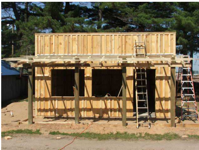
Saturday June 9 th 2007, front porch roof installed.
